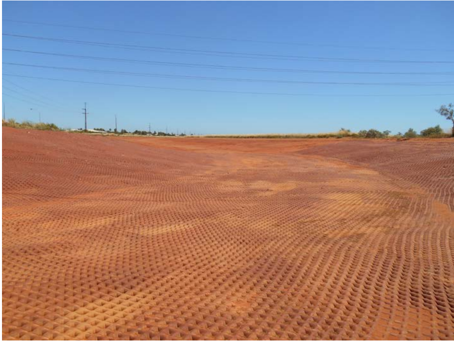
Plate 1 Constructed Drainage Channel
