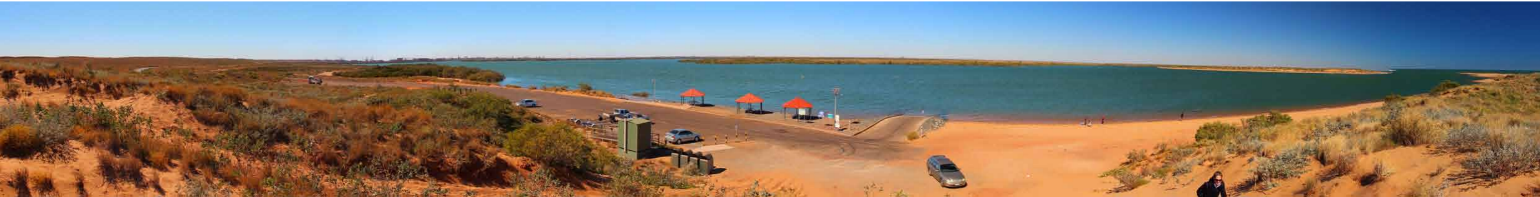
View over the existing boat ramp facilities at Finucane Island, looking South East
