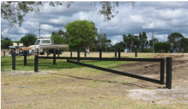
Lockable gates to entry points to control seasonal access
