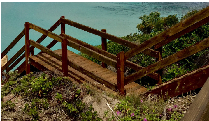
Timber or steel stairs to steep access points
