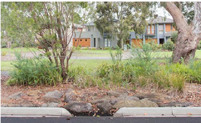
Installing breaks within kerbs and directing stormwater to trees and planting.
