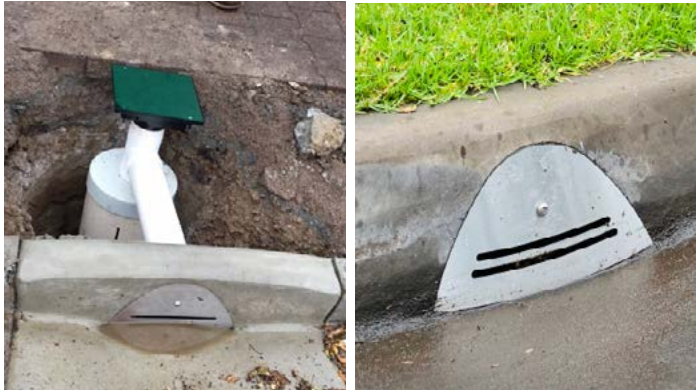
Tree inlets shown being installed into existing kerbs (left) and shown when fully installed (right).
