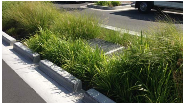
Installing breaks within kerbs in planted medians and roadside verges to recharge soil moisture.
