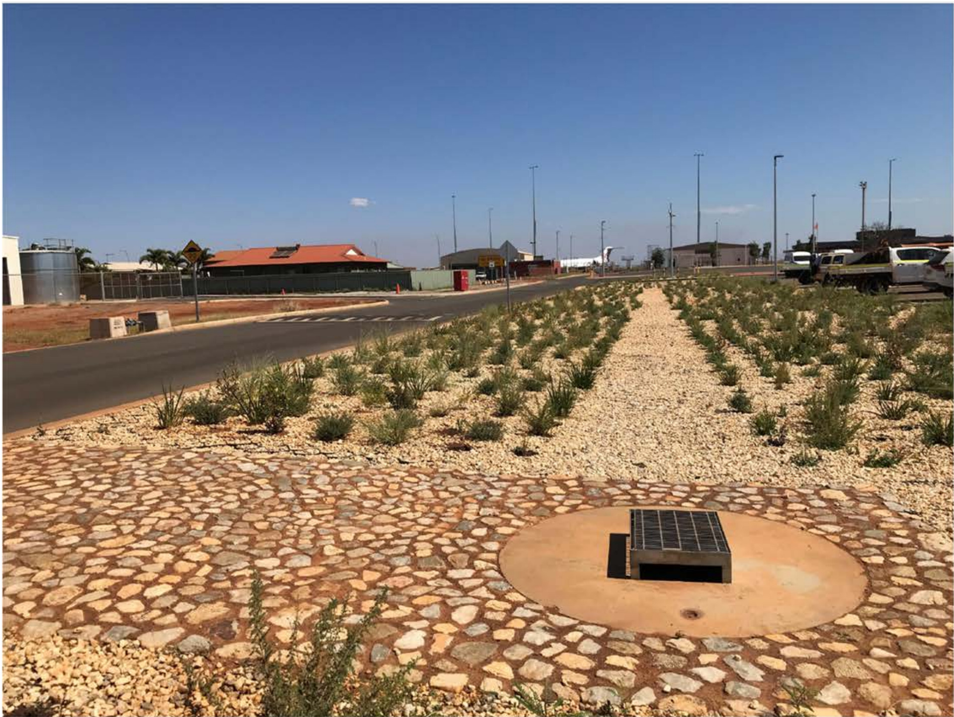
Figure 9: A swale and discharge point protected with a mixture of ground stabilisation matting, landscaping, cemented rock pitching and larger stones (Port Hedland)
