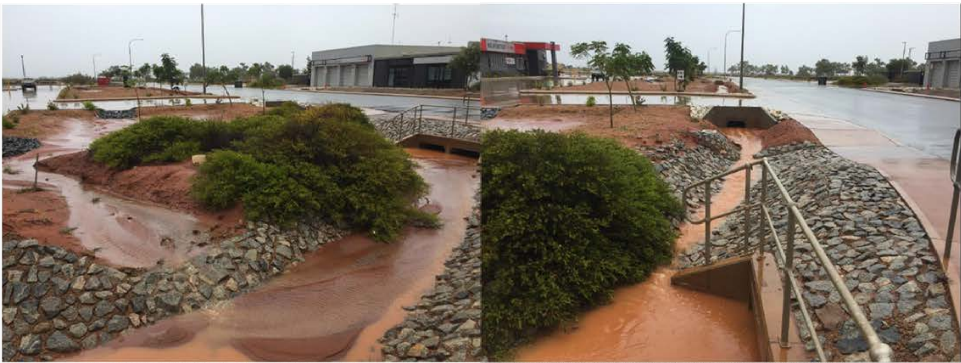
Figure 5: Silt from private property has entered a public drain, will reduce its effectiveness and require cleaning out (Kingsford Smith).
