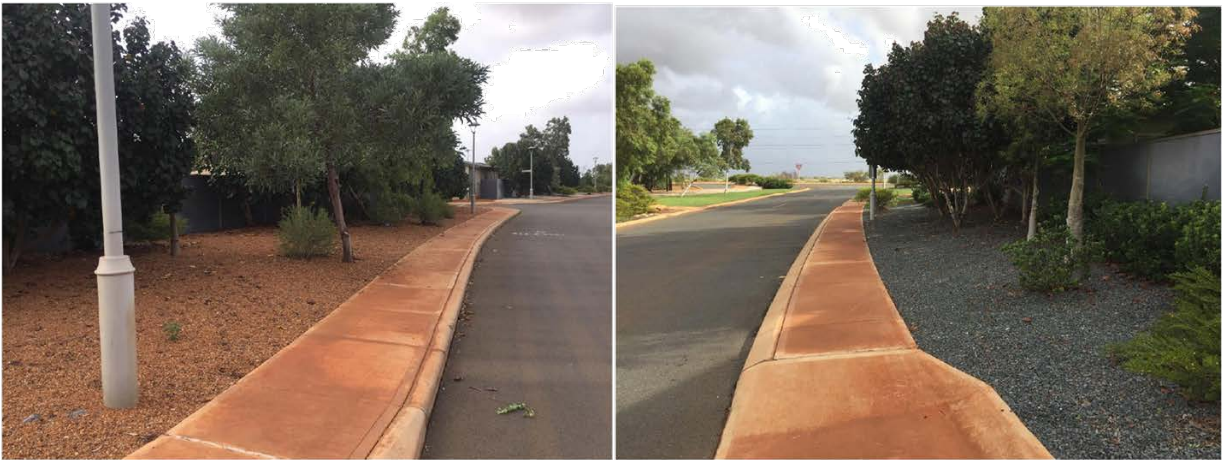
Figure 6: Verges that have been installed with 20-50mm river shingle or blue metal and to a depth of 100mm after experiencing 290mm of rain over three days (South Hedland)
