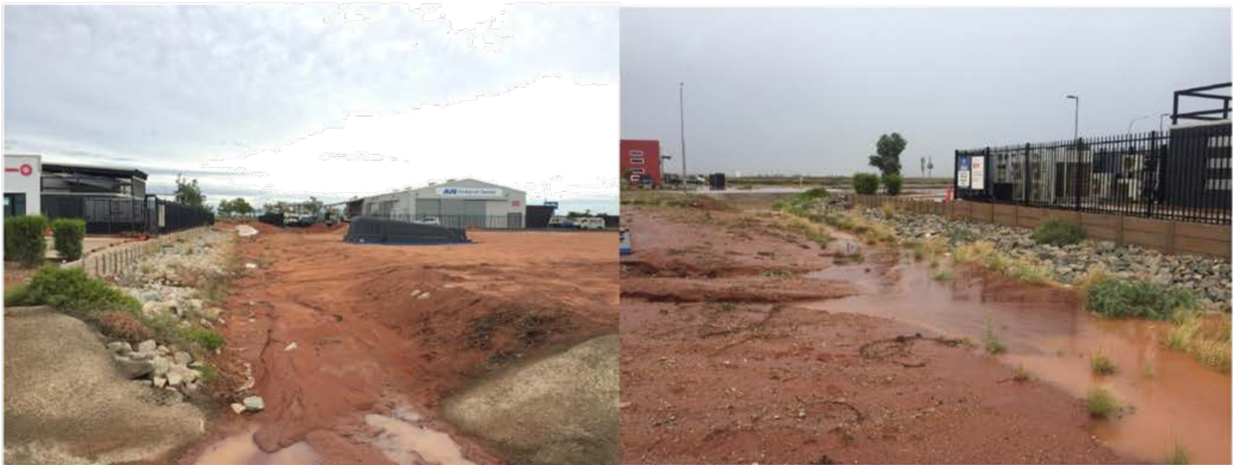
Figure 4: A public drain that has become blocked from eroded pindan (Kingsford Smith).
