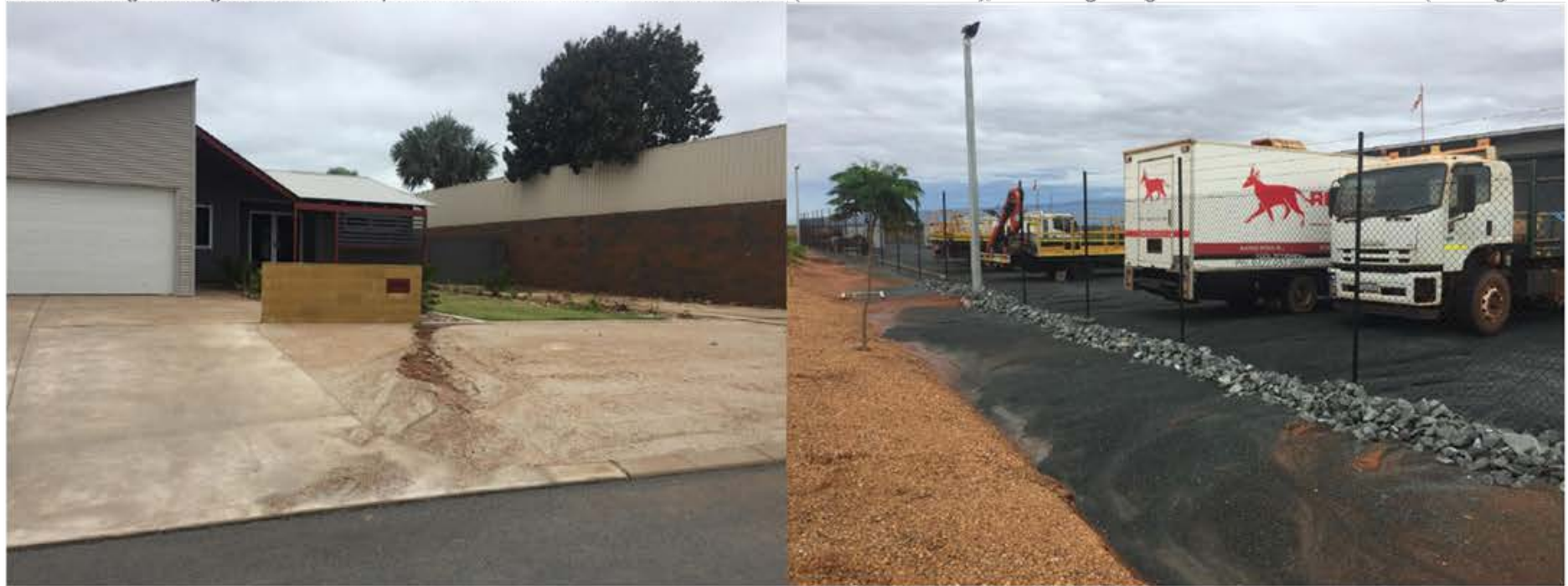
Figure 3: Verges and yards consisting of fines, such as cracker dust, are highly prone to erosion (left Port Hedland, right Kingsford Smith).
