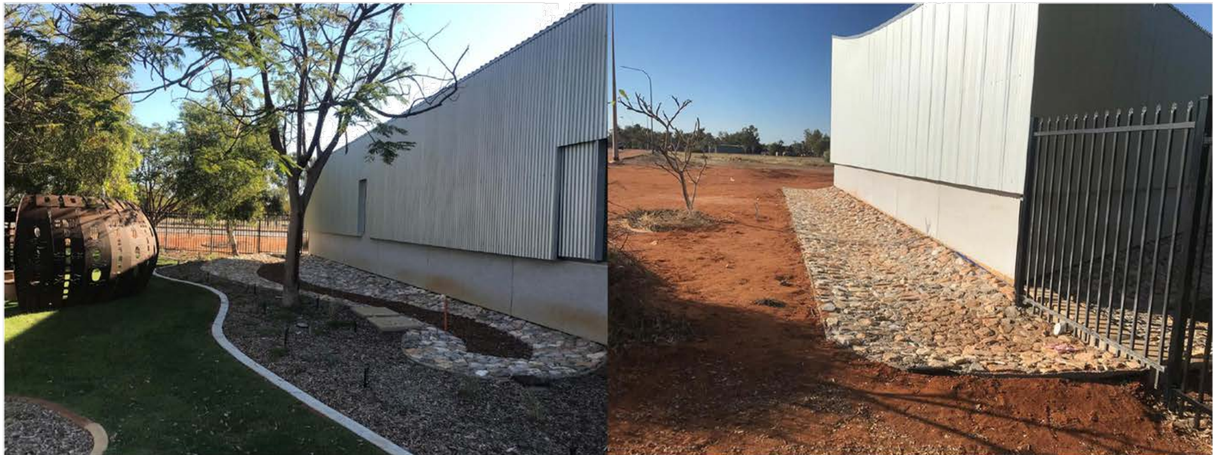
Figure 10: Left, a detention basin that captures this roof's runoff prior to discharging excess water into the public drainage system. Right, the discharge point into the public drainage system (South Hedland)
