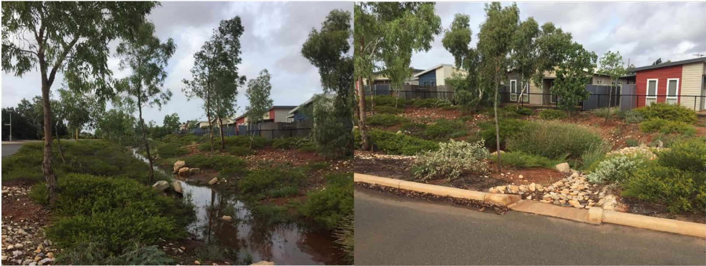
Figure 8: A vegetated swale (left) and cemented rock pitched discharge point (right). These have held their form, transported water away efficiently and do not require cleaning out or regrading despite 290mm of rain over three days (South Hedland).
