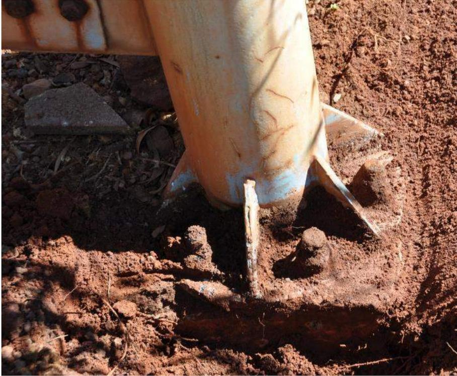
Figure 8: Column base connection to foundation
