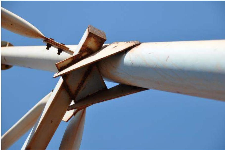
**Figure 11: Underside of connection between beam B1 and column**
