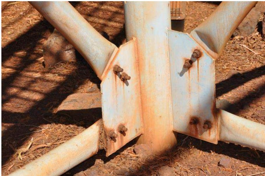
**Figure 13: Connection between struts and braces at base of column**
