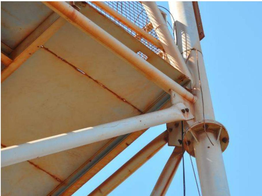
Figure 9: Column splice and strut and brace connections
