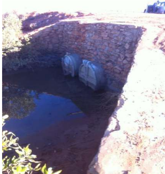
Plate 1 Culverts under Cooke Point Drive
