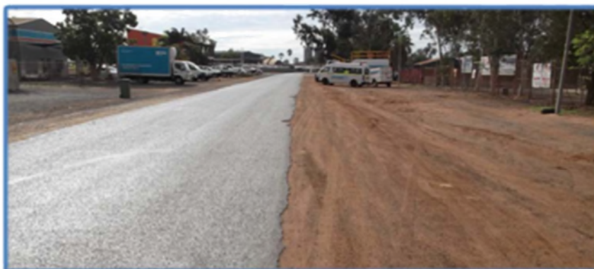
Yanana Street – Edge break up, no swale, verge parking
