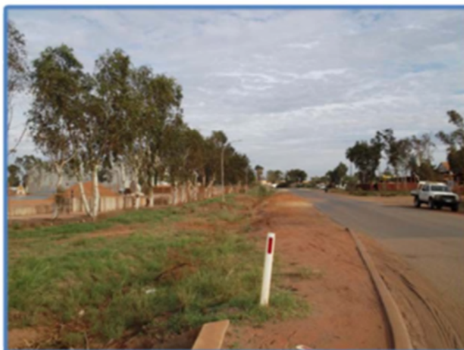
Yanana Street – Edge break up, no swale, verge parking
