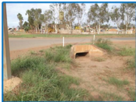
Peawah Street – Headwall close to corner, growth within swale (Area 1)
