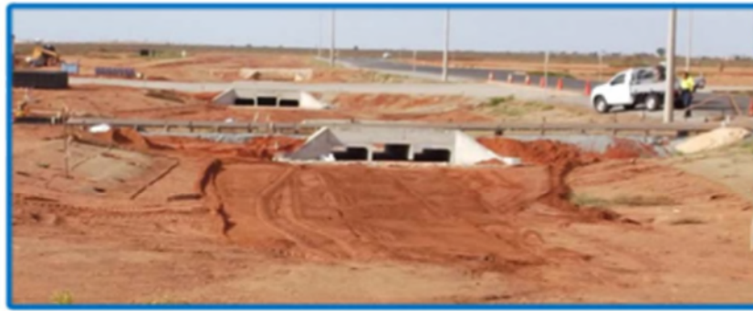
Hematite Drive – New development drainage swales and cross-over (Area 4)
