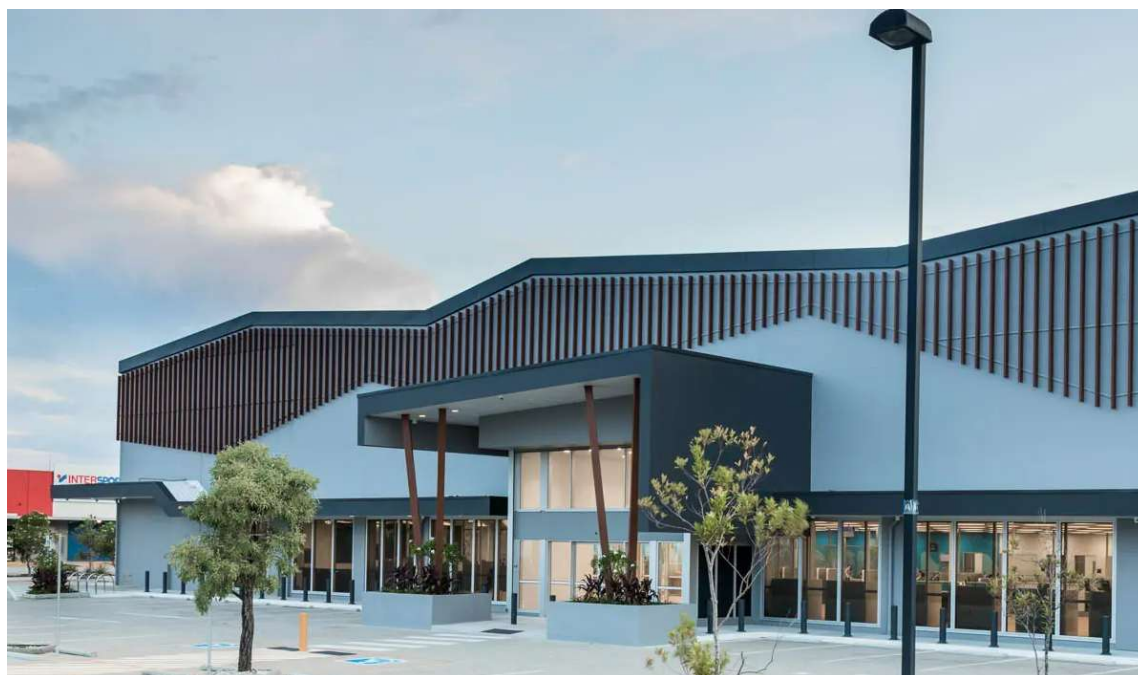
Figure 2: Example of how variation in height and roof articulation can be used on the façade to create visual interest. (Image: HomeCo Cairns, Tomkins Commercial, 2021)
