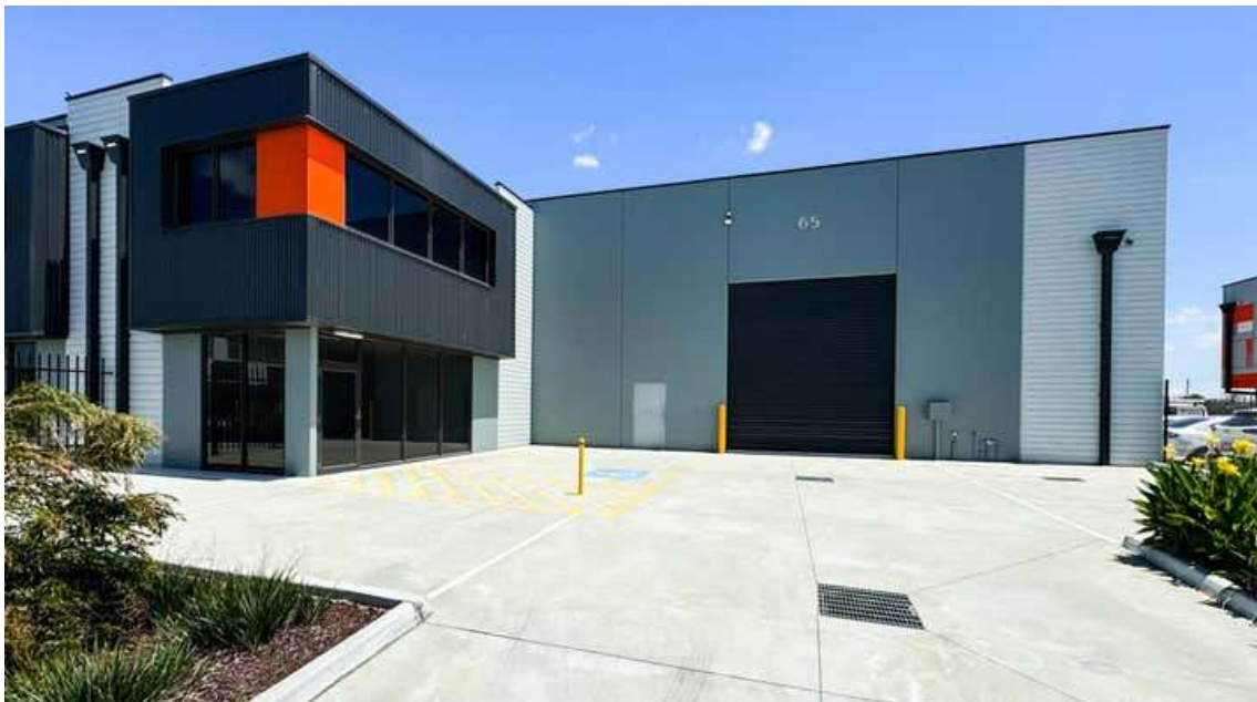
Figure 9 – Example of clear separation between visitor and service vehicle areas and use of materials to highlight the office area. (Image: Cranbourne West, Cameron)
