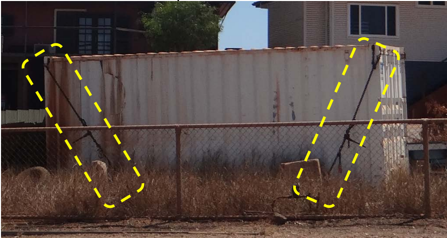
Not permitted in Scenario B, C, D, G, H & I – tie down chains and straps
