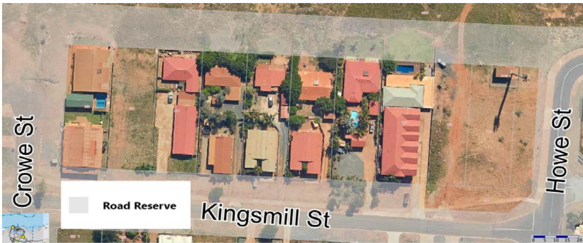
Fig 1 – Example of Kingsmill St Encroaching Property Boundaries
