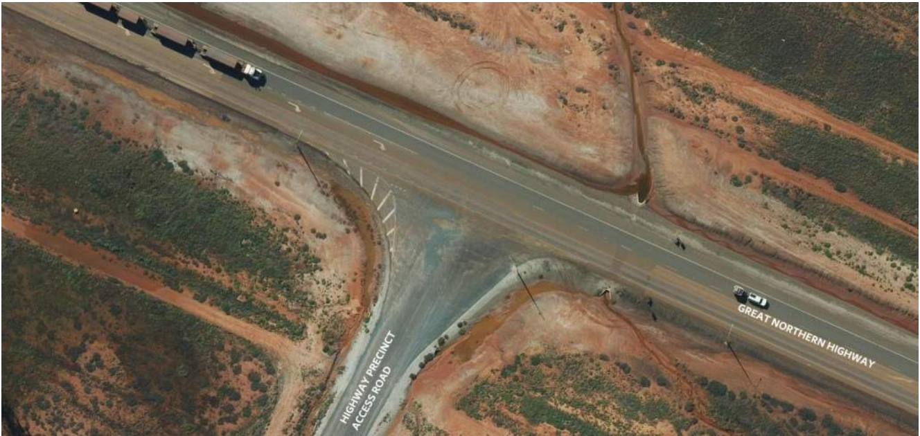
Figure 22 Existing Great Northern Highway and Highway Precinct Access Road intersection layout (aerial image source: MetroMap)
