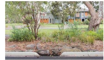
Installing breaks within kerbs and directing stormwater to trees and planting.
