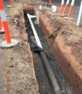
Infiltration systems consist of infiltration trenches, swales and basins, and are designed to retain a certain volume of stormwater runoff. The stormwater recharges surrounding soils adjacent trees and reduces runoff volumes.
