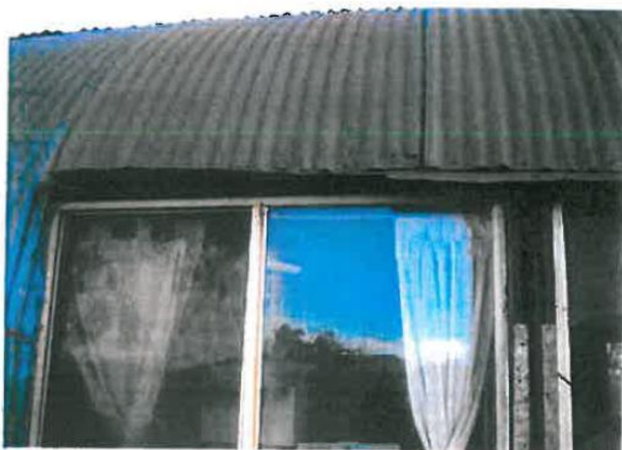
Front detail showing aluminium framed windows.
