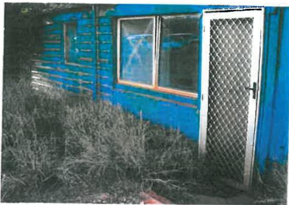
Detail of northeast corner of the extension
