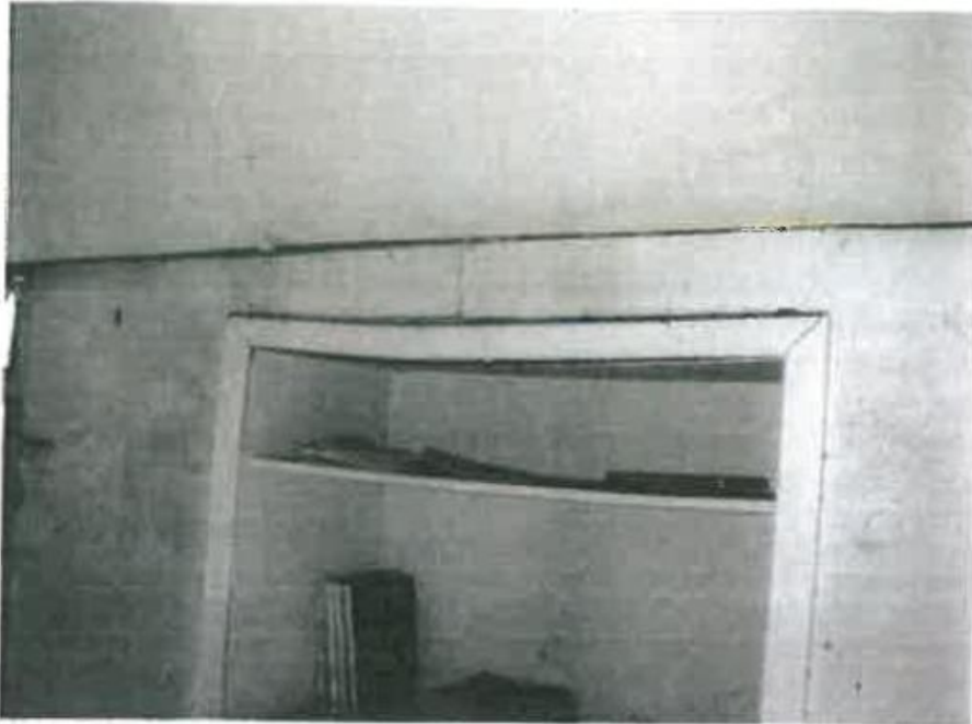
Interior: kitchen, chimney alcove on the street frontage.
