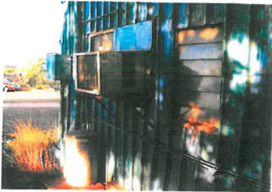
Detail of the wall at the east end showing interventions.
