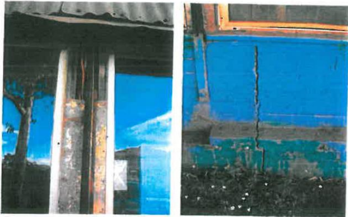
Front detail showing adhoc nature of the Interventions; structural cracking.
