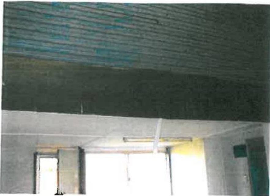
Interior: View looking into the north extension where the wall has been removed, showing ceiling levels and linings.
