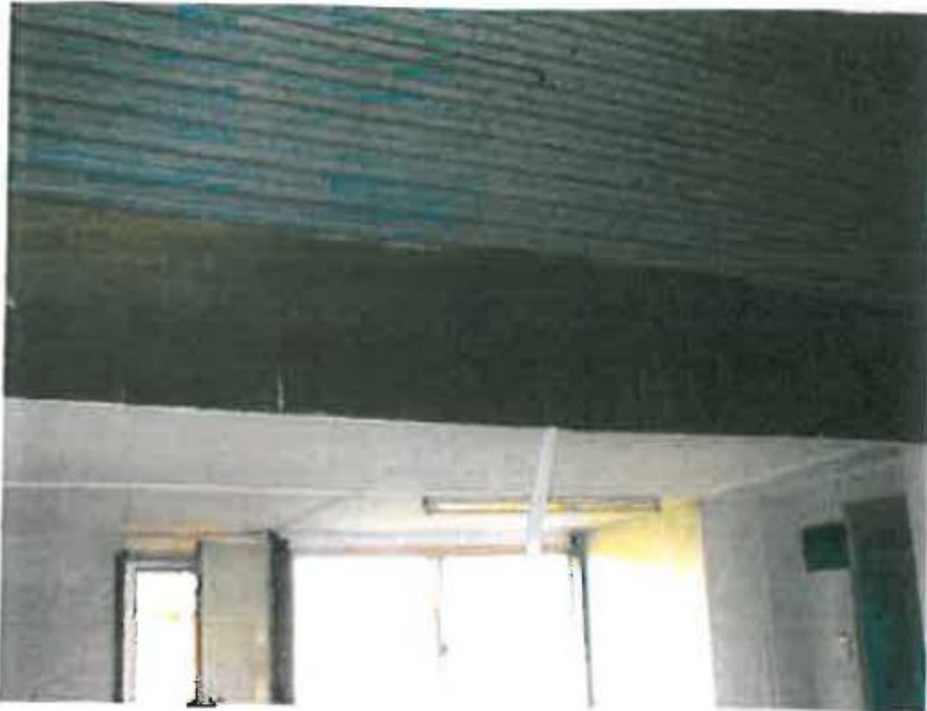
Interior: View looking into the north extension where the wall has been removed, showing ceiling levels and linings.
