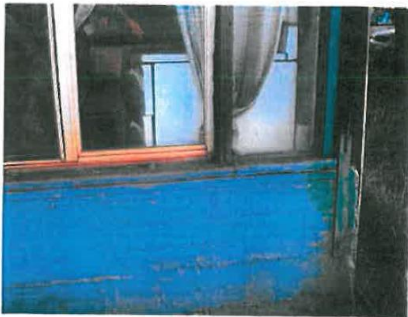
Front of southeast corner (kitchen) showing off form concrete and steel bracing detail.
