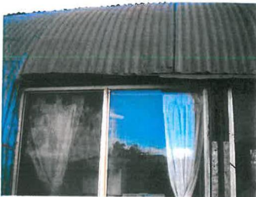
Front detail showing aluminium framed windows.
