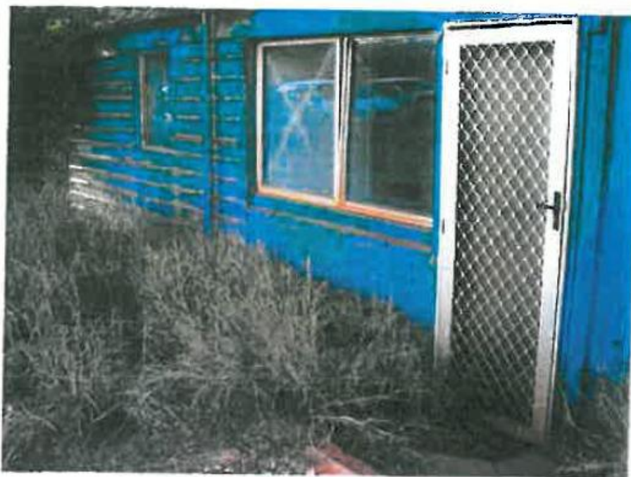
Detail of northeast corner of the extension
