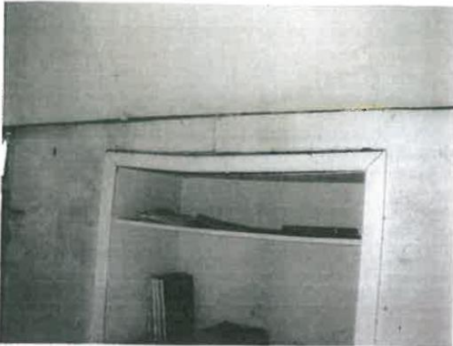
Interior: kitchen, chimney alcove on the street frontage.
