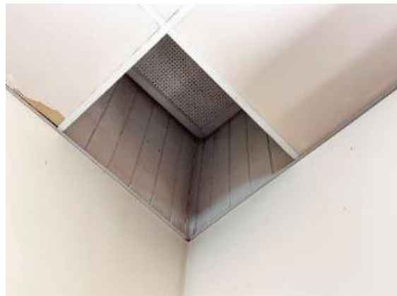
Figure 56: View through acoustic tile ceiling towards original level of ceiling
