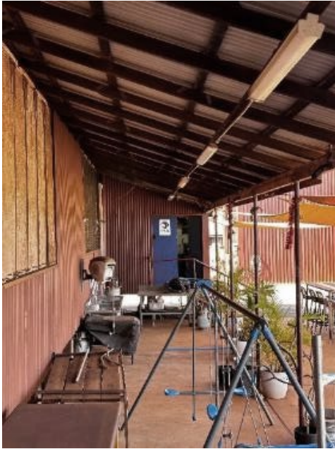
Figure 36: View along rear elevation to Marine Rescue office entrance
