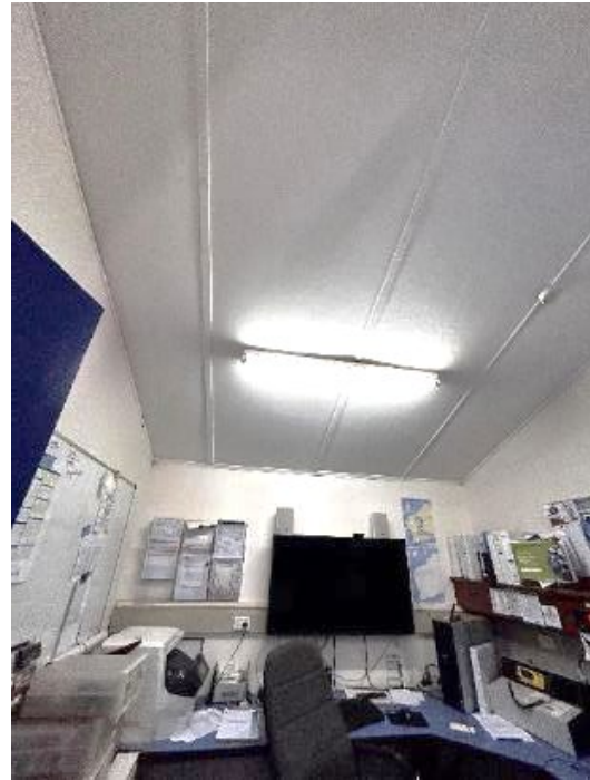
Figure 64: Ceiling to Radio Room
