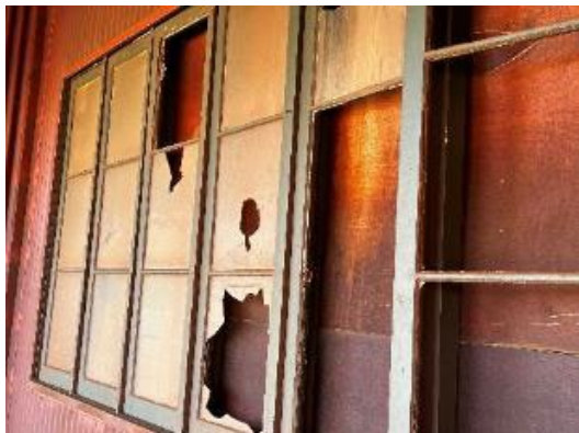
Figure 65: Broken glazing
