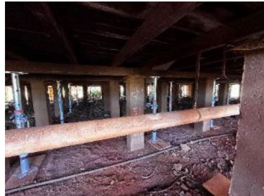
Figure 80: Acrow props underneath building
