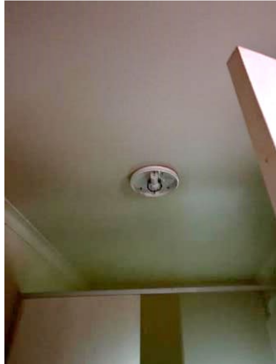
Figure 50: Plasterboard ceiling to toilet
