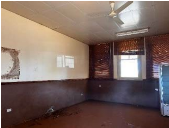
Figure 52: Original classroom (Main Hall No. 2)
