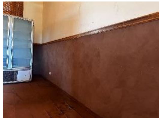
Figure 90: Non-original wall finish in Main Hall 2 (original school room)
