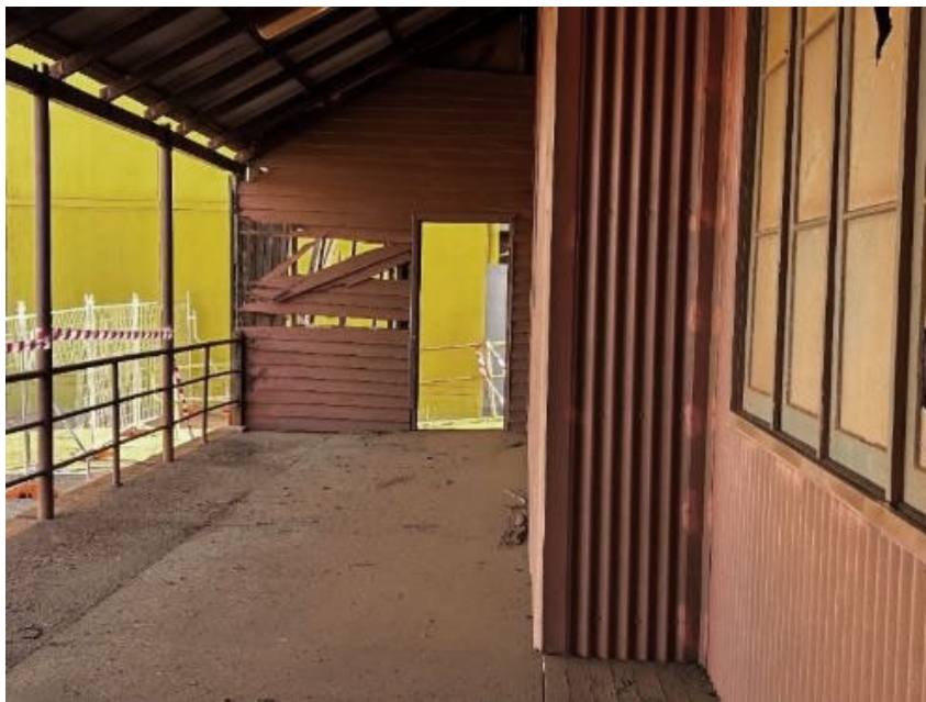
Figure 37: View along rear elevation towards original section of the school
