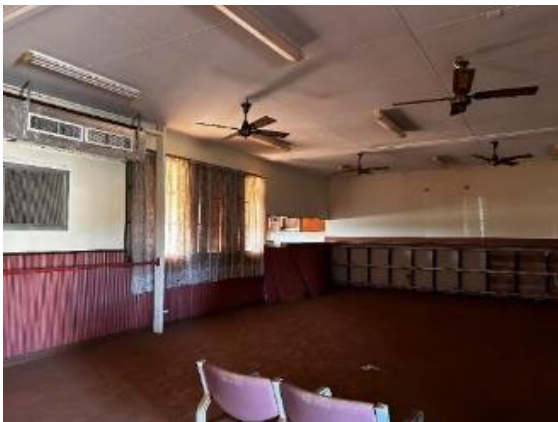
Figure 39: Main Hall No. 1 looking towards kitchen in far corner
