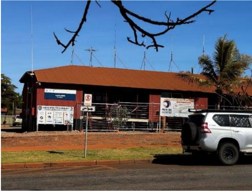
Figure 28: South western end of the former Port Hedland State School building, now used as Marine Rescue office
