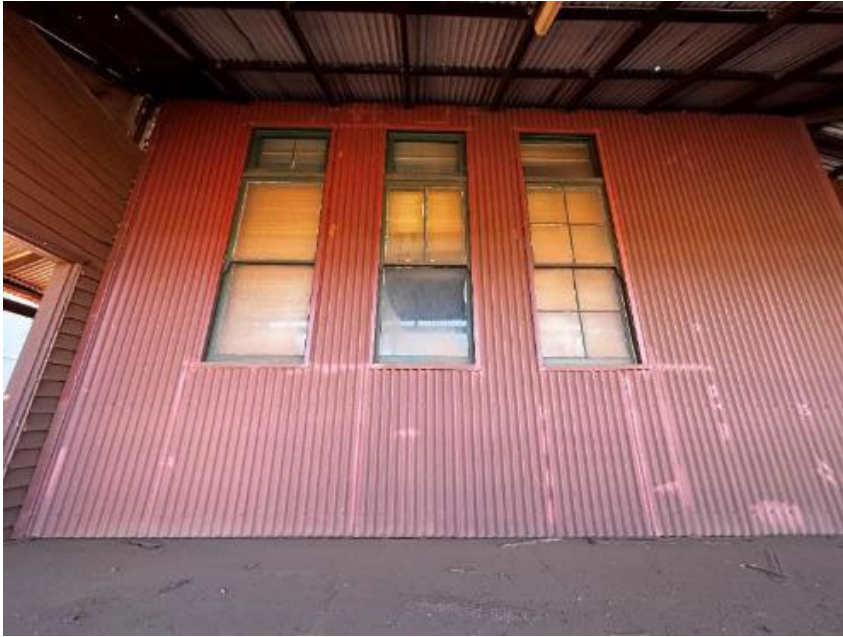
Figure 34: Windows to original section of school building
