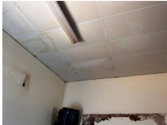
Figure 54: Acoustic tile ceiling
