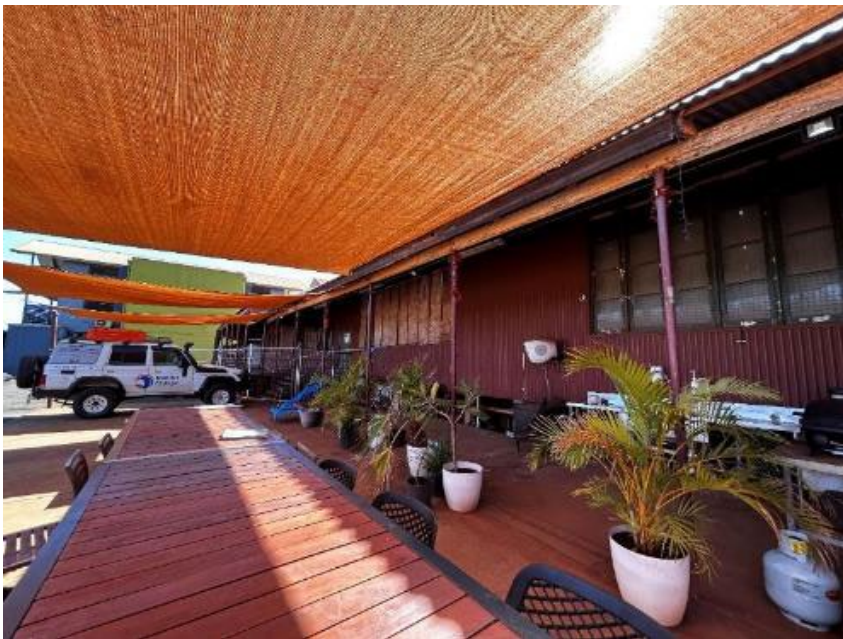
Figure 35: View along rear elevation
