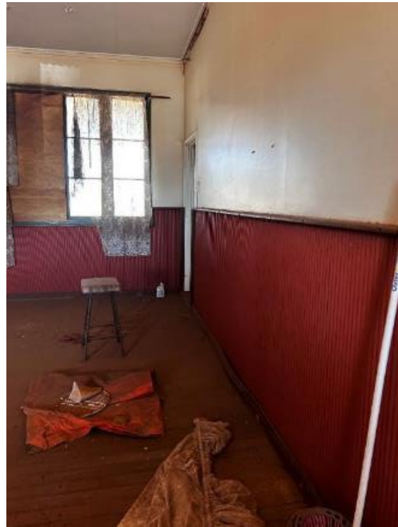
Figure 47: Custom orb dado along north-west wall of Main Hall No. 1
