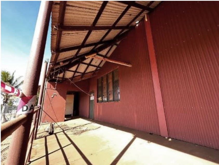
Figure 30: View along front verandah
