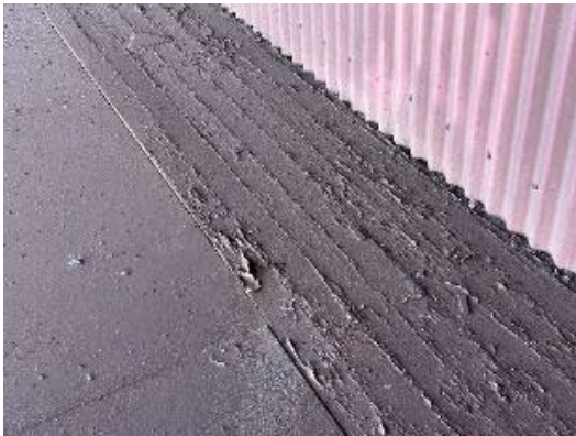
Figure 71: Deteriorating verandah timbers
