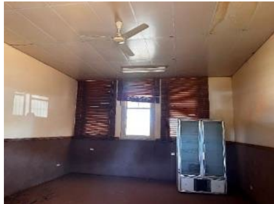
Figure 51: Original classroom (Main Hall No. 2)
