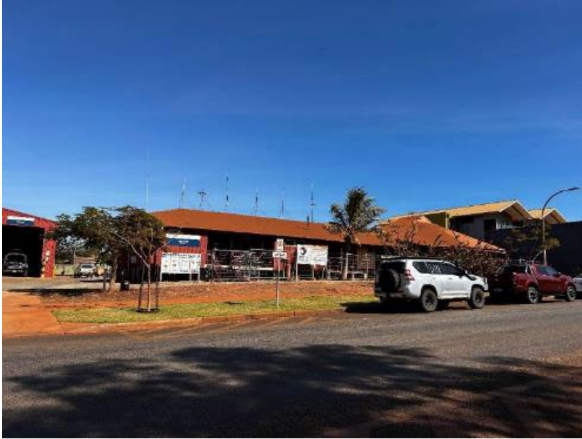
Figure 24: Lot 869 Tower Street, Gwalia – façade
