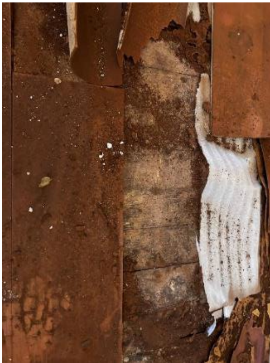
Figure 53: Timber floor under existing floor lining
