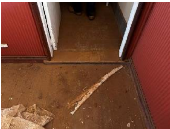
Figure 46: Stepped access into toilets
