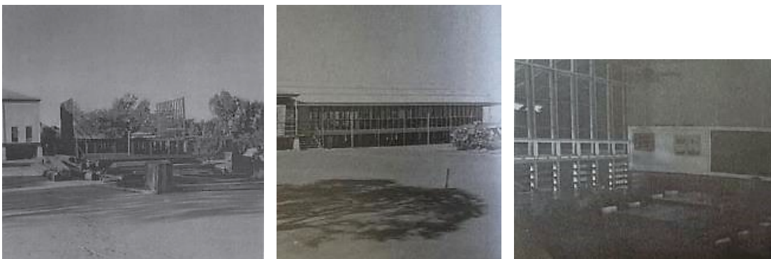
Figure 18 Construction of the two new classrooms Courtesy 'Through Dusty Eyes', p. 42.
