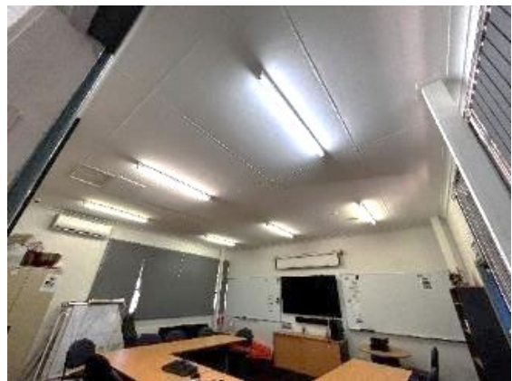
Figure 61: Ceiling to Meeting Room
