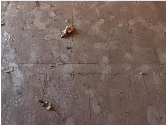
Figure 45: Timber floor Main Hall No. 1
