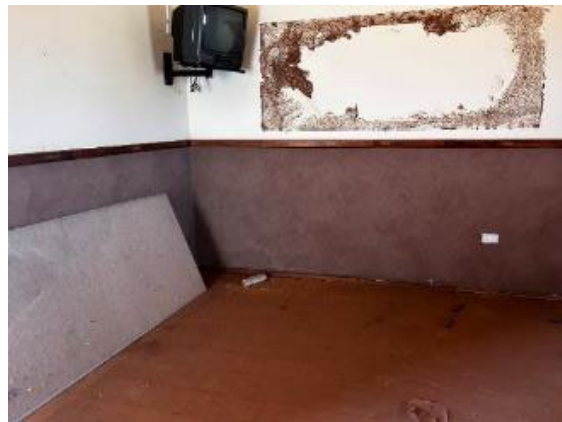
Figure 55: Dado around the walls of the original classroom
