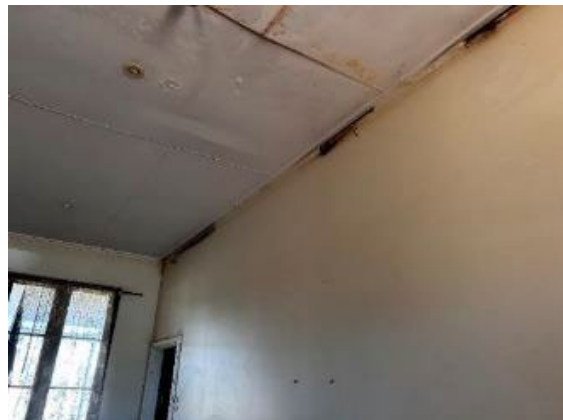
Figure 48: Upper section of north-west wall and asbestos sheet ceiling lining
