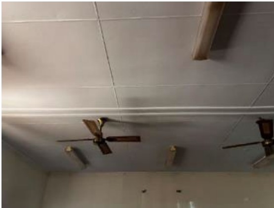
Figure 44: Ceiling in Main Hall No. 1
