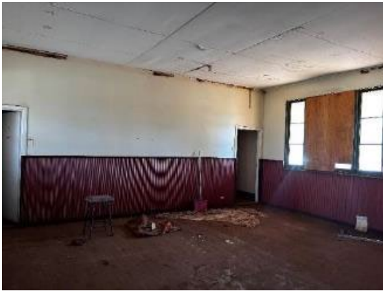
Figure 38: Main Hall No. 1 looking towards toilets
