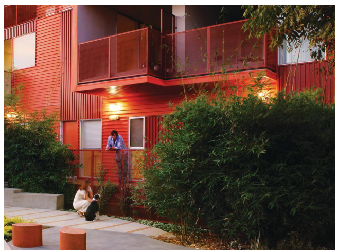
A good example of a raised ground floor balcony adjacent to the public realm, providing a balance between privacy and relationship to street.
