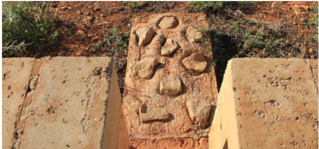
An example of controlling and minimising overflow and flooding through simple detailing, in this instance it allows for overflow from a small
