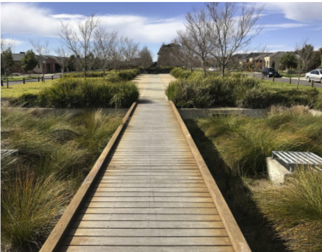
Ensuring larger drainage swales can be crossed via dedicated pedestrian paths or elevated walkways.
