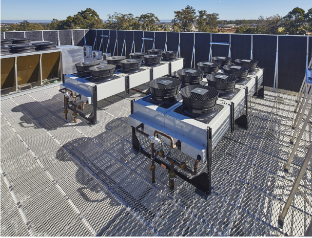
Acoustic screens for roof services and air conditioning units can further reduce noise.
