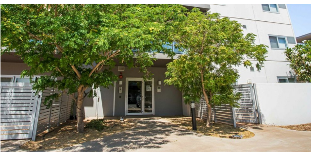
Recessed pedestrian entries supported by shade, and co-located with entries to private front yards.
