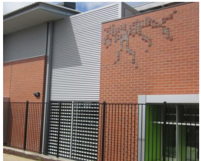
Examples of service enclosures and screening treatments designed as an integral part of the overall development.
