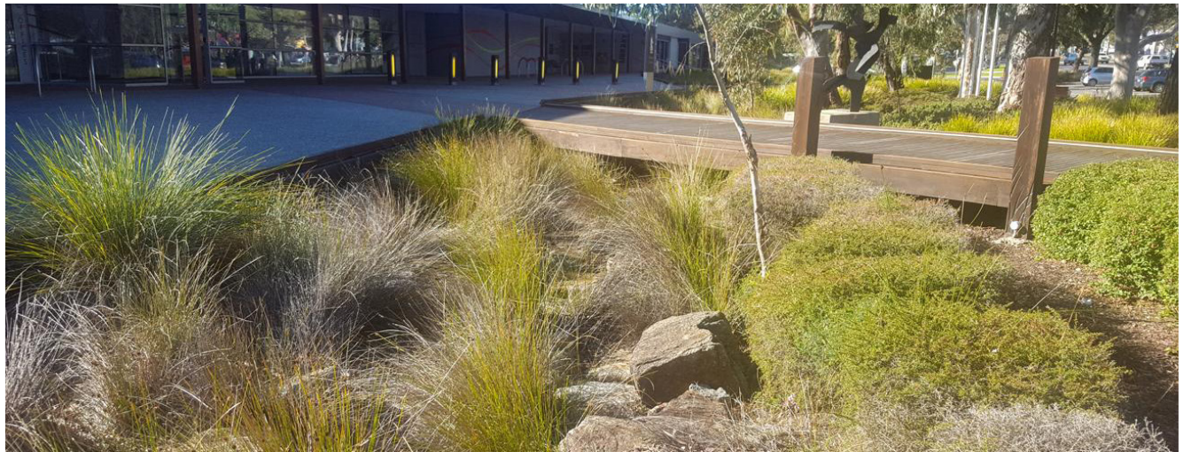
Large swales and Water Sensitive Urban Design gardens can deal with more intense overland flow events.
