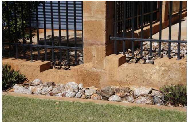
An example of controlling and minimising overflow and flooding through simple detailing, in this instance it allows for overflow from a small
