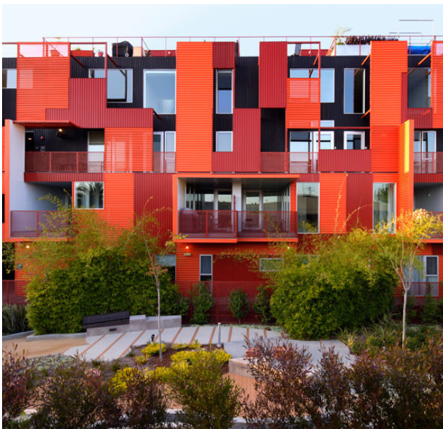
An example of a building facade that provides articulation and screening devices to openings and upper level balconies.
