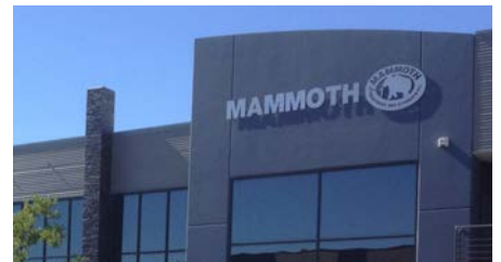
Signage integrated into the fabric of the building.
